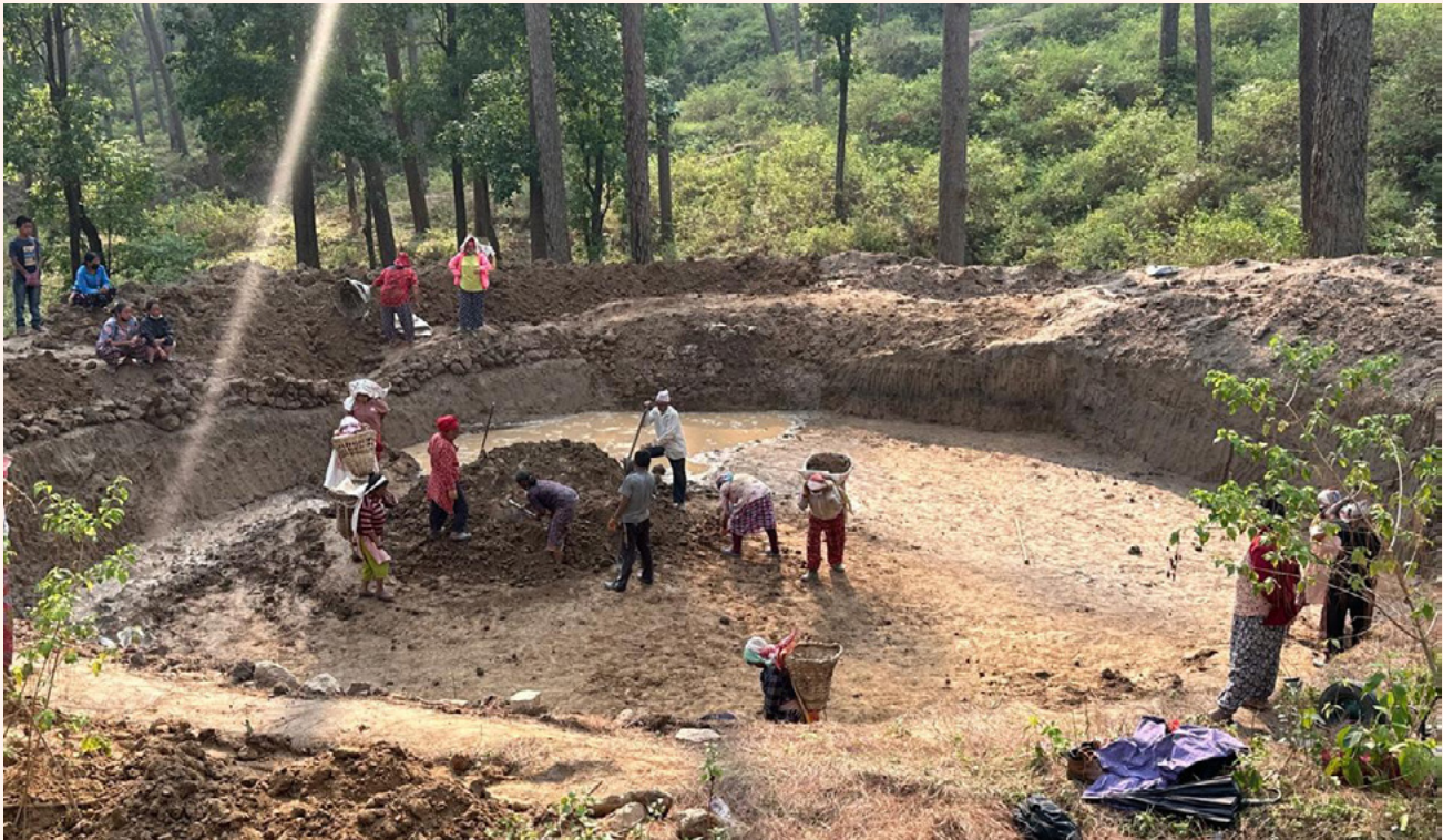
Workers constructing water recharge pond in Dhankuta Municipality, Nepal
