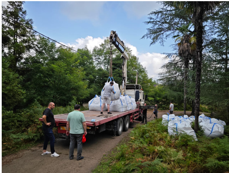
Fig.2 Loading bags on the truck to transport for safe storage
