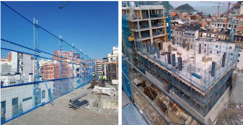
Image 4. Combined design solution of a construction net and railing
