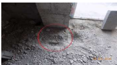
Fig. 5. Local open r/c floor slab (outlined in red)
