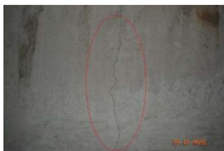
Fig. 11. Cracks in beamless monolithic r/c floor slab (outlined in red)
