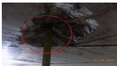
Fig. 6. Measuring of r/c floor slab protective layer thickness (outlined in red)
