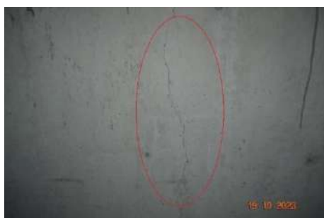
Fig. 10. Cracks in beamless monolithic r/c floor slab (outlined in red)
