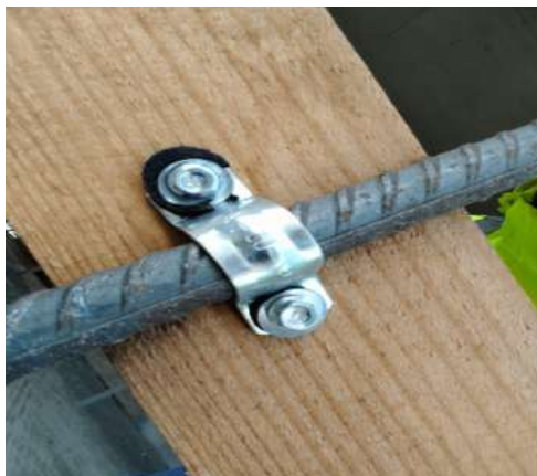
Image 1. Guardrail plank clamp and reinforcement support
