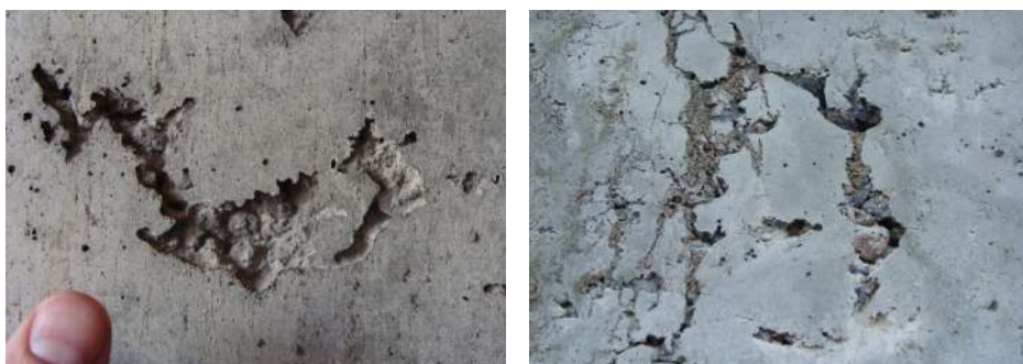
Fig.2. Macro-sized voids on the concrete surface
