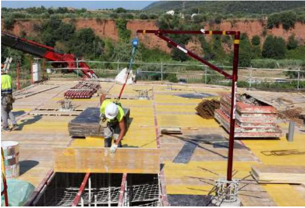
Image 2. Working at height using guardrails and fall arrest equipment
