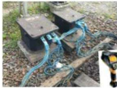
Fig.5. Throttle-transformer jumpers heating video control
