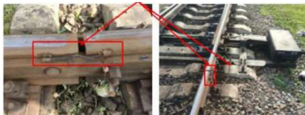
Fig.4-control of duplicated (welded) couplings
