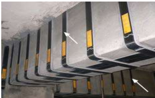
Fig. 16. Reinforcement of the Bearing Coils of the Reinforced Concrete Bridge Structure with Carbon Fiber-Reinforced Plastic
