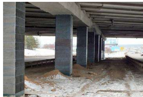
Fig. 17. Reinforcement of the Middle Supports of the Reinforced Concrete Bridge with Carbon Fiber Tape FibArm
