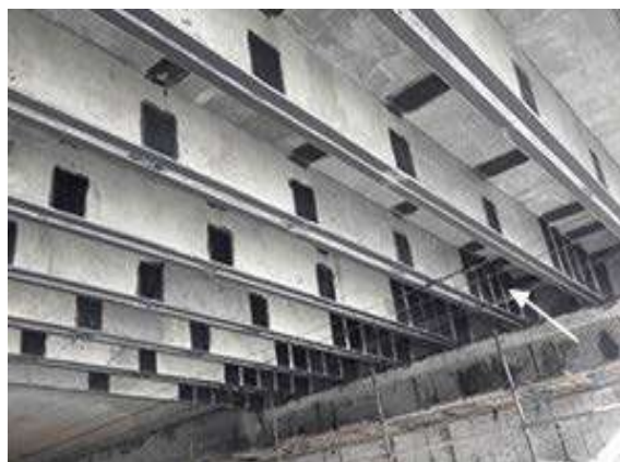
Fig. 14. Reinforcement of Longitudinal Bearing Coils with Carbon Fiber Tape
