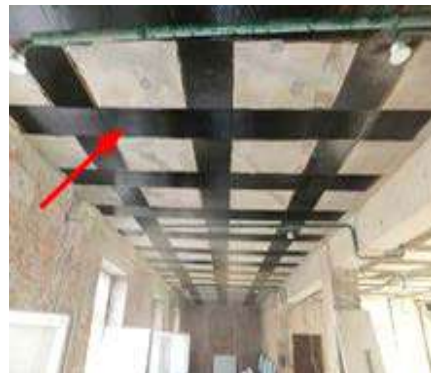
Fig. 11. Reinforcement of Reinforced Concrete Roofing from the Bottom with Carbon Fiber Tape
