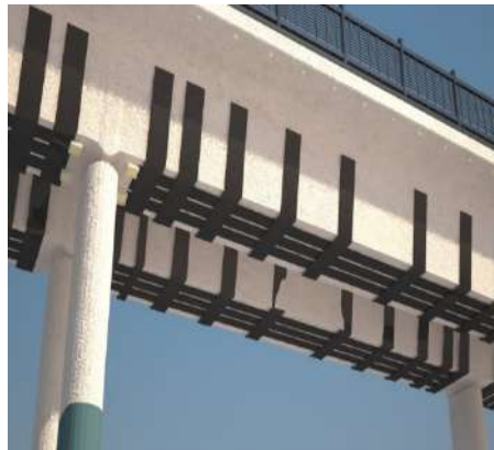
Fig. 13. Reinforcement of the Structure of the Bridge with Carbon Composite Tape
