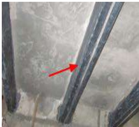
Fig. 12. Reinforcement of the Plate with Carbon Composite
