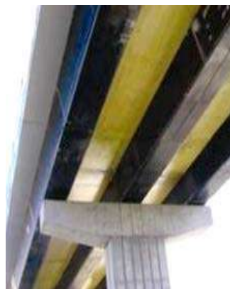
Fig. 15. Reinforcement of the Tongitudinal Beams of the Road Bridge with Carbon Fiber Tape
