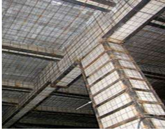
Fig. 11.7. Eeinfforced Concrete Coils and Columns Reinforcement With Casing
