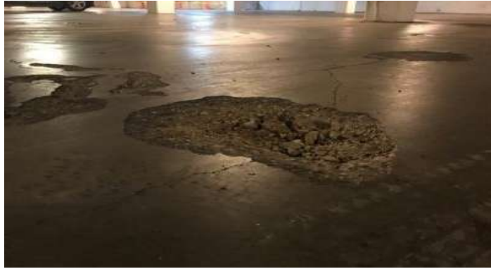
Figure 9. Damage caused by corrosion of reinforced concrete parking structures.
