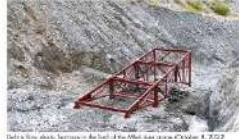
During the construction of the new water management system.
